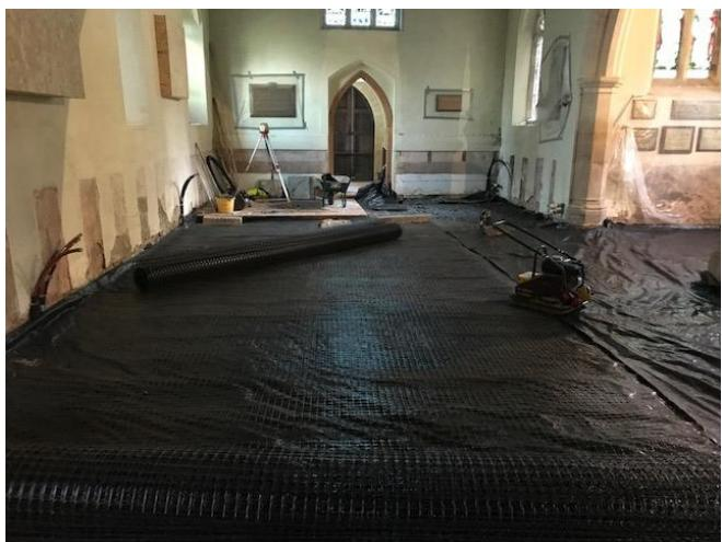
The next picture is looking towards west door of the Nave with the gravel in position and the next layer of geotextile material in position. In the foreground is the heavy duty net that the heating pipes will be clipped to. The picture below again shows this material place.
