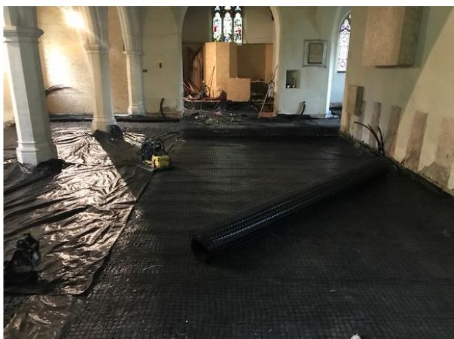
There's still a bit of sorting out to do around the vaults and in the Chancel where a concrete base has to be placed ready to take the stone step into the enlarged area of the Sanctuary. Once that's complete then the under-floor heating pipes can be placed in position. Already the pipework is in place going down beneath the Organ Chamber into the cellar below the Vestry. Here the connections can be made to the boiler which is in the Priest's Vestry just above the cellar.
