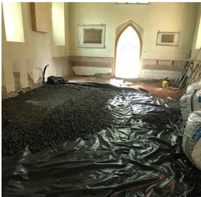
Following on from last week the first picture shows the glass insulating layer being put in place over the geotextile material.
